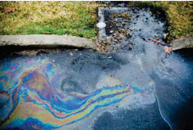
Typical diffuse urban pollution concentrated at a conventional gully.
