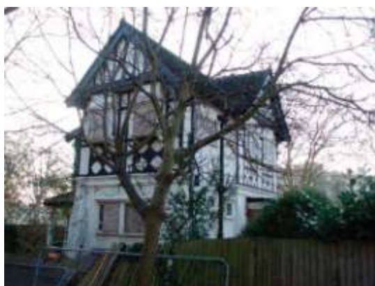
Derelict buildings provide potential for bat roosts.
