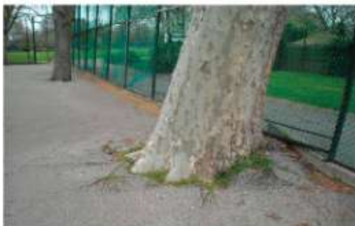
Fencing conflicts with mature trees
