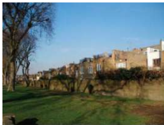
Boundary wall and adjoining land could be used to establish habitats
