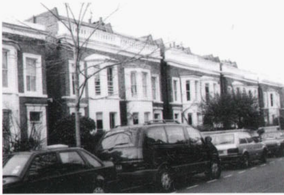
Nos. 20-26 Ashchurch Grove, locally listed.
