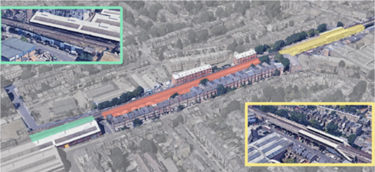
Image 6: Location of arches 192-219(East) and 212-240 (west) between Goldhawk Road and Trussley Road
