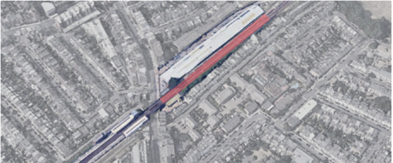
Image 16: Location of arches 1-4 and Parsons Green Commercial Estate/ Depot, 33-39 Parsons Green
