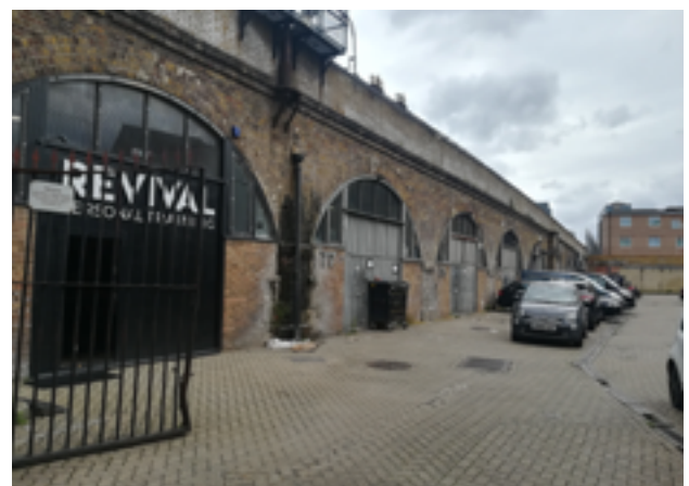
Photo 9: Glenthorne Mews arches to the South of the track
