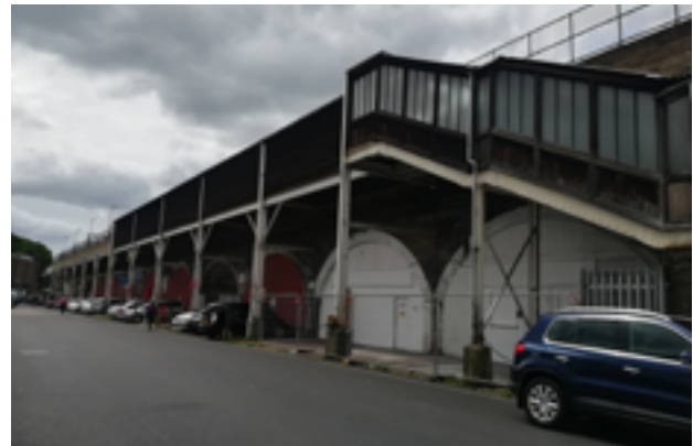
Photo 5: Arches to the East of the railway arches on Wells Road
