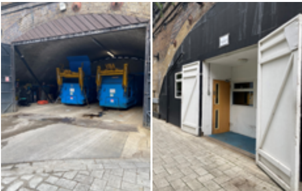
Photo 18: Arches used as refuse storage (left) and office (right)
