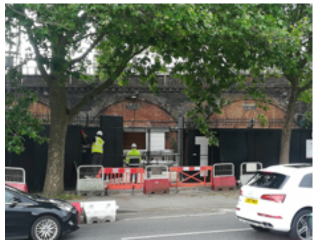
Photo 2: Arches in the former BBC Television Centre
