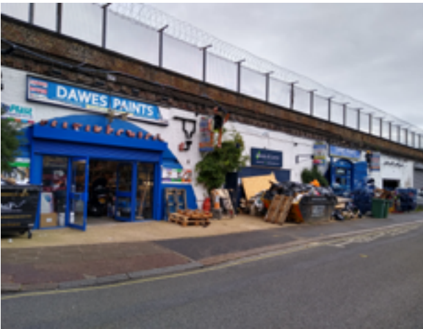
Photo 6: Arches 234-240 to the West of the track in Trussley Road
