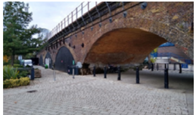
Photo 19: Pedestrian open arch and occupied arches to the South of the track
