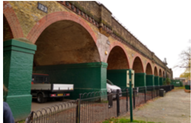
Photo 11: Arches in use by the Council as storage
