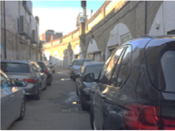
Photo 15: Arches fronting the rear of the premises on the New King's Road
