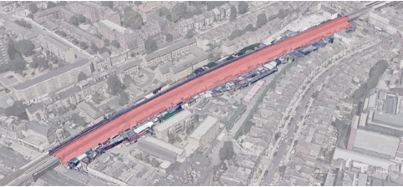
Image 5: Location of arches 155-191 between Uxbridge Road forming part of Shepherd's Bush Market
