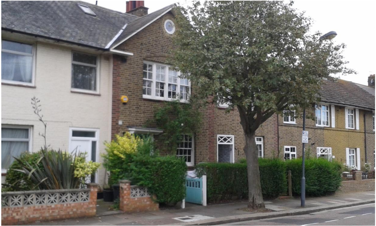
No. 129 Braybrook Street - gable roof with oriel window. Unfortunately No. 127 has been painted, the porch has been filled in and multi-paned windows have been lost. The original diamond lattice in the porch is visible in No. 129.
