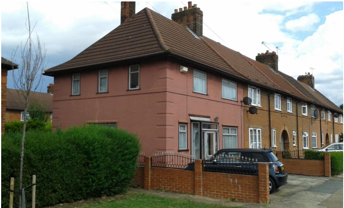
Painted facades at No.24 Daffodil Street together with a modern glazed porch and inappropriate replacement windows diminish the uniformity of the terrace. Fortunately, the string course and the brick work relief detail on the corner are still visible under the paint.
