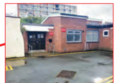
Lytton Residents Hall Lytton Estate, North End Crescent London W14 8TE Thursday 2.30-4.30pm
