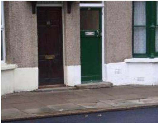
**Figure 4.3-8 Example of Raised Property Thresholds**
