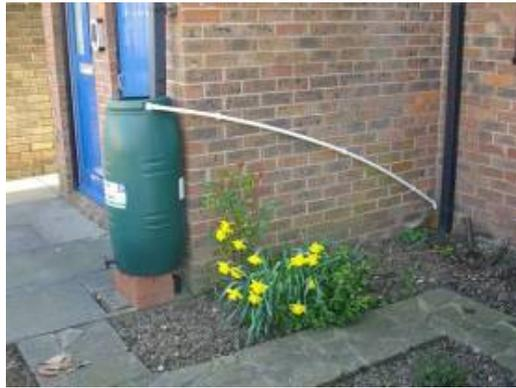
**Figure 4.3-7 Example of a 100L Water Butt Retrofitted to Existing Development**
