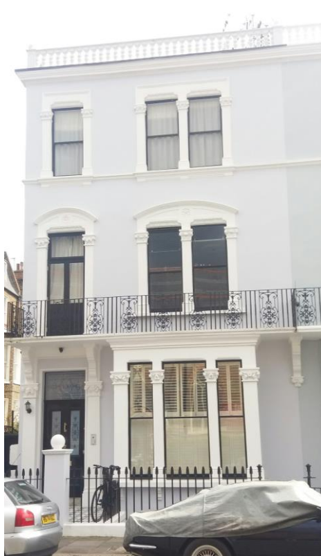
Bottle balustrade parapet and ornate iron balustrade at No. 100 Masbro Road.
