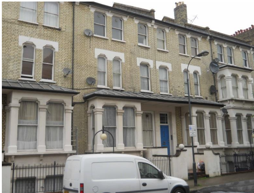
Lakeside Road, gault bricks and stucco bays found on Nos. 32 to 106 (even) and 43 to 97 (odd).
