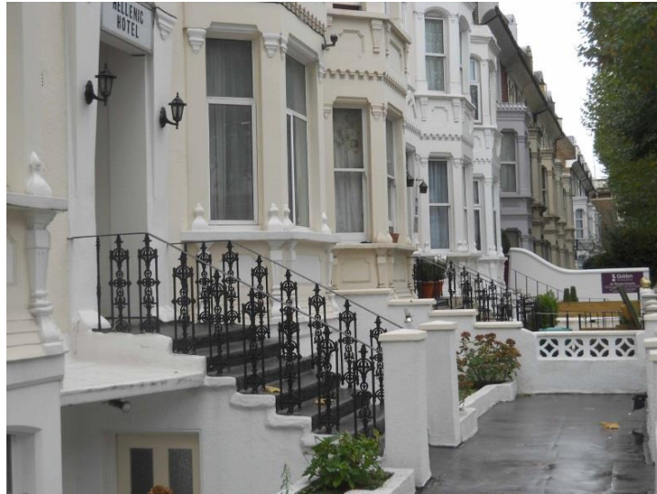
Nos. 77-85 Shepherd's Bush Road have vase like pilasters under the sills and finials above. Ornate railings remain on some.
