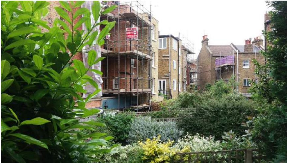
Nos. 51-67 Bolingbroke Road. The pattern of closet wings at the rear of the terrace is clearly visible from Milson Road.
