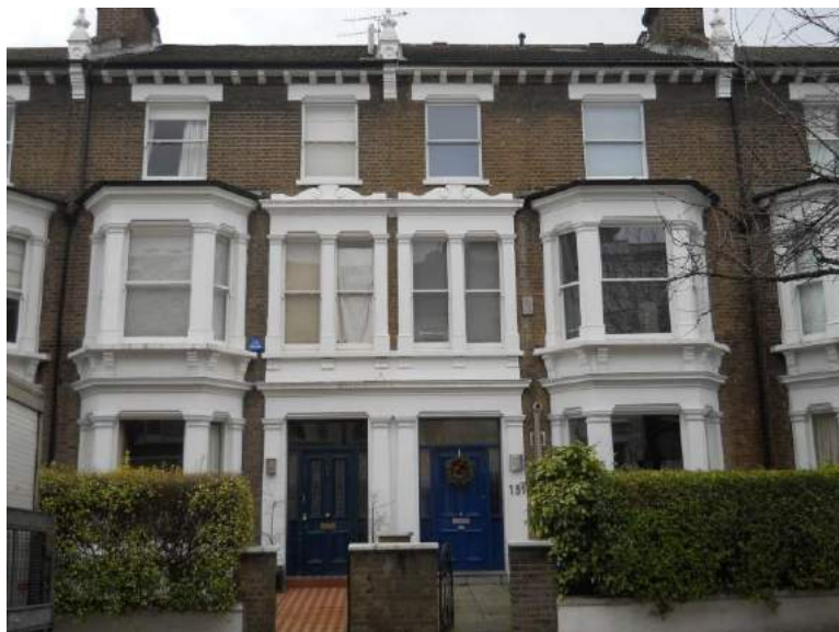
Paired windows above the entrances with stucco scrolled pediments Nos. 145 to 161 Blythe Road.
