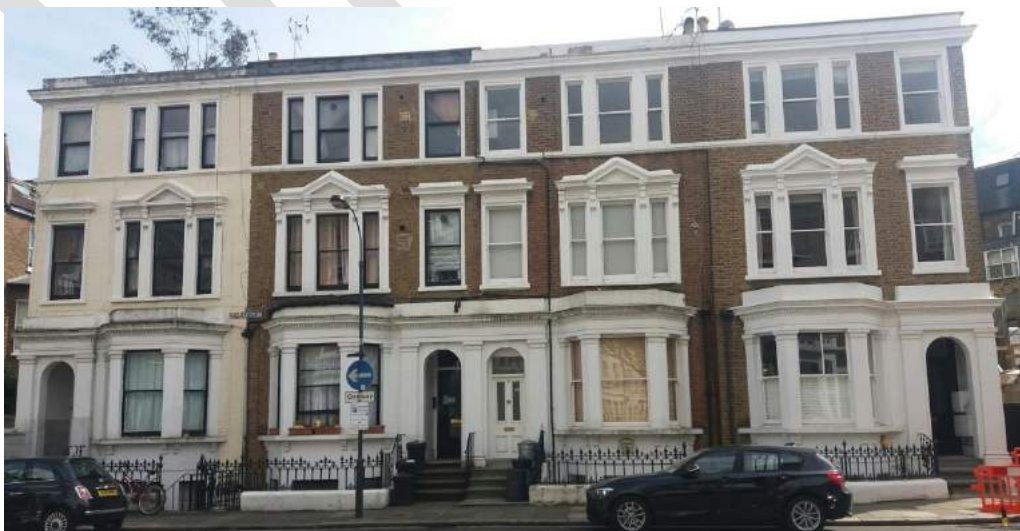
Nos. 1-7 Hazlitt Road. First floor windows with pediments that are typical in this character area.
