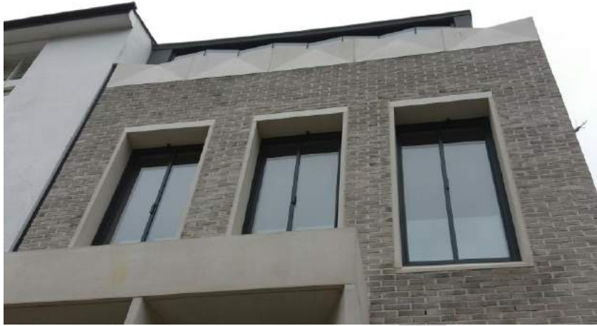
No. 121 Milson Road. Attractive details include deep window reveals, faceted parapet and upper storey glazing.
