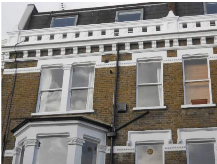
Elaborate stucco parapets on Nos. 1-21 and 2 -24 Bolingbroke Road with prominent later additional storeys.
