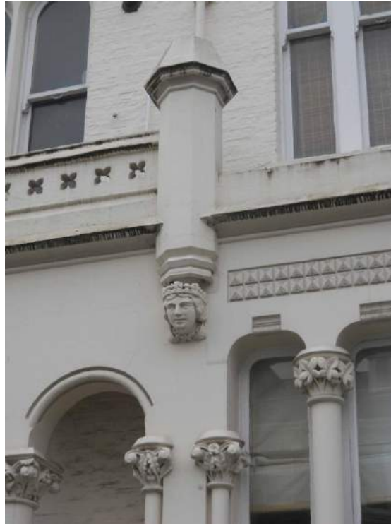
Masks, finials and slender columns with capitals. Nos. 1 to 43 and 3 to 33 Sinclair Road.
