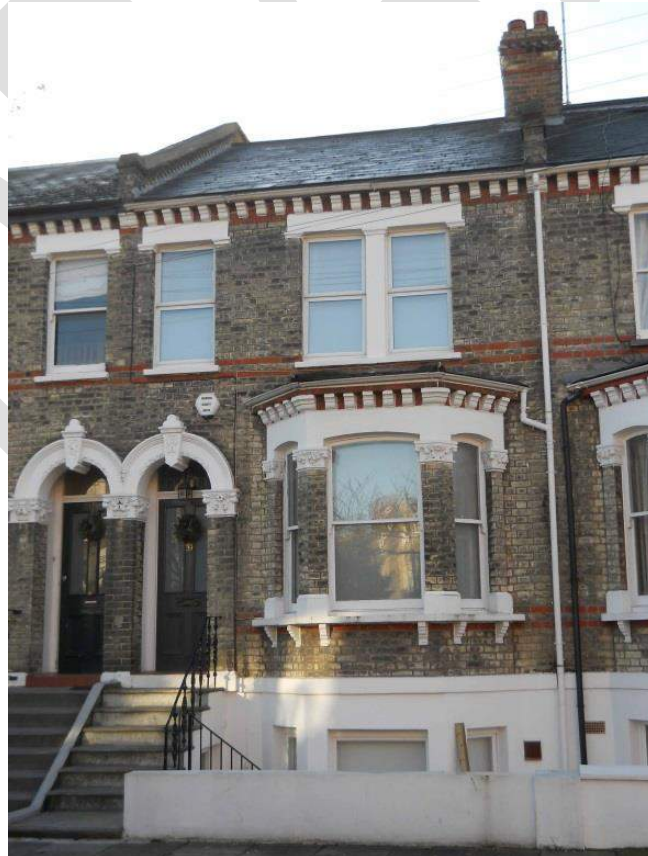
Nos. 25 to 45 Irving Road. Gault brick facades with red brick string courses. Note the distinct modillions under the eaves.
