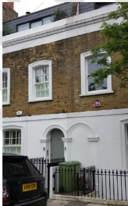
Infilled porch, no. 53 Faroe Road.
