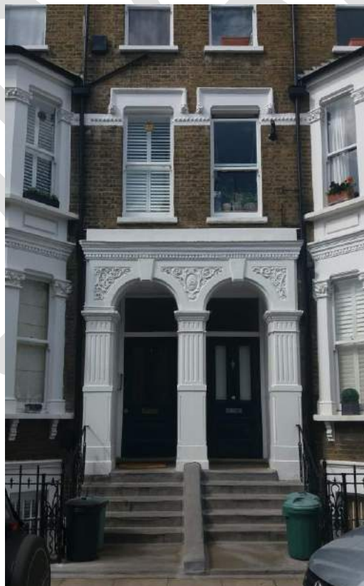
Nos. 2-24 Bolingbroke Road. Richly detailed stucco porches.
