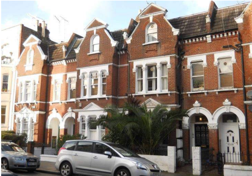
Houses in Addison Gardens, Nos. 142 to 148. Richly detailed facades are further enhanced by planting in front gardens.
