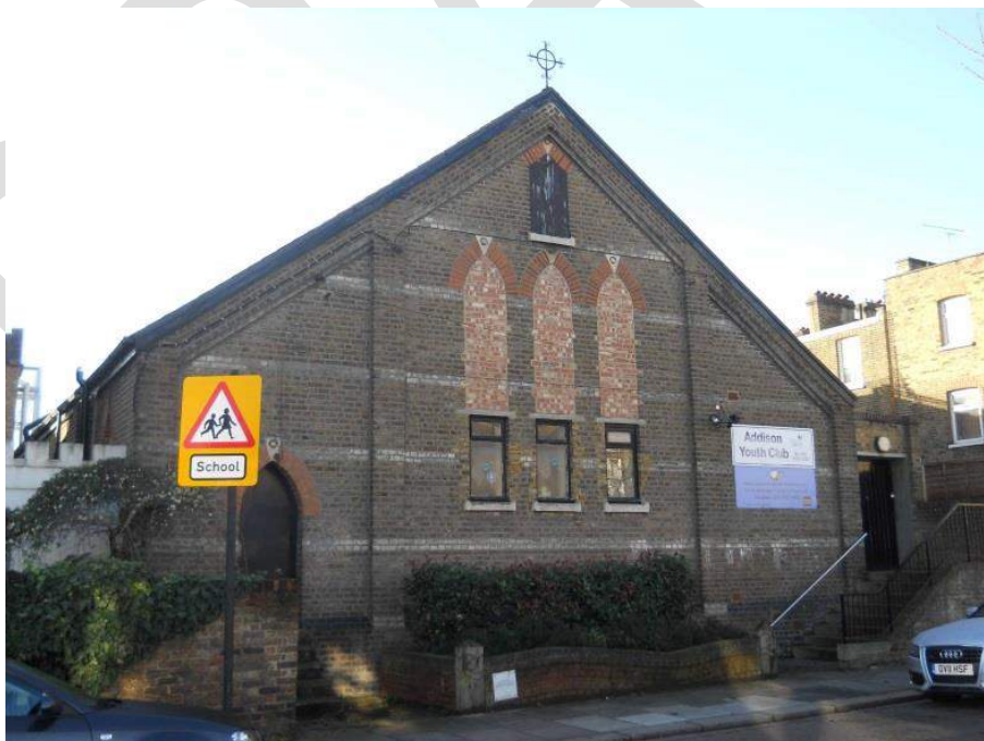
Bricking up of windows on Addison Boys Club has harmed the appearance of this elevation on Redan Street.
