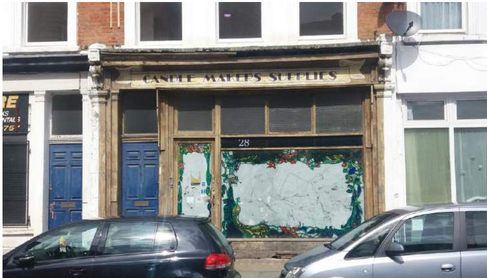
Well-proportioned shopfront at no. 28 Blythe Road in need of some repair.
