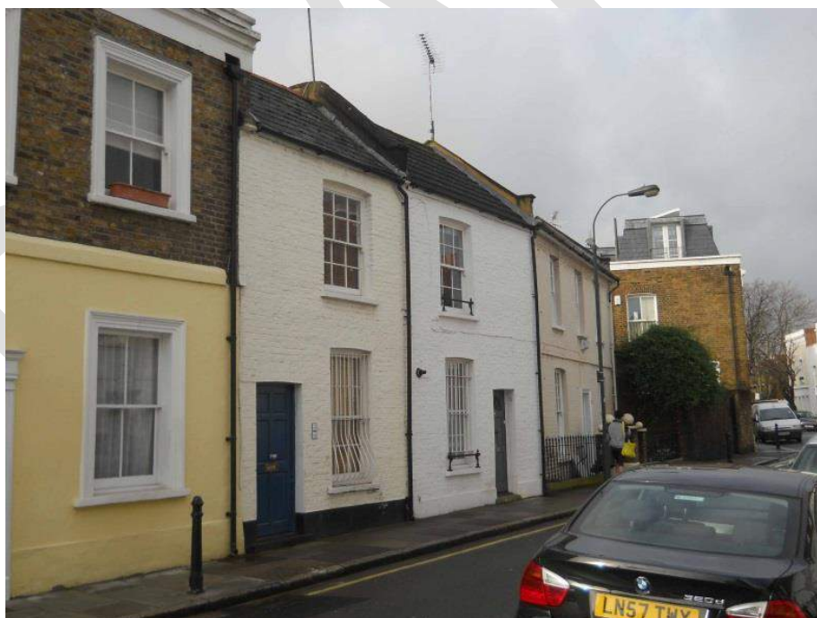
Nos. 42 to 48 (left) Milson Road.
