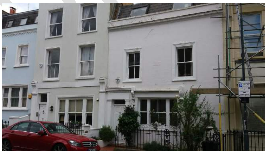
Nos. 71 and 73 Milson Road as they are now with retained pilasters and console brackets and cornices (no. 73 only).
