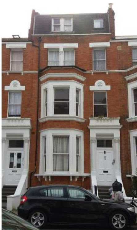
No. 92 Netherwood Road.
