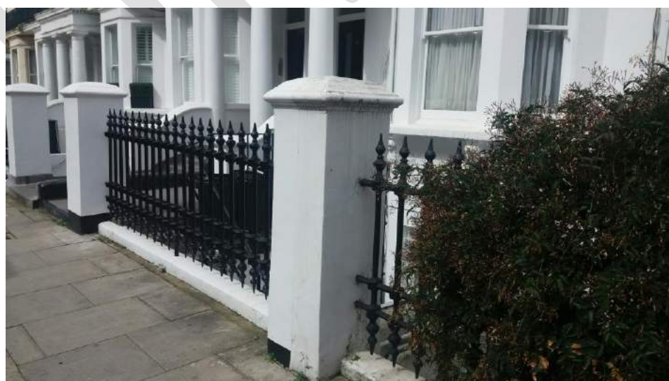
Original iron railings and piers are largely intact, Maclise Road.
