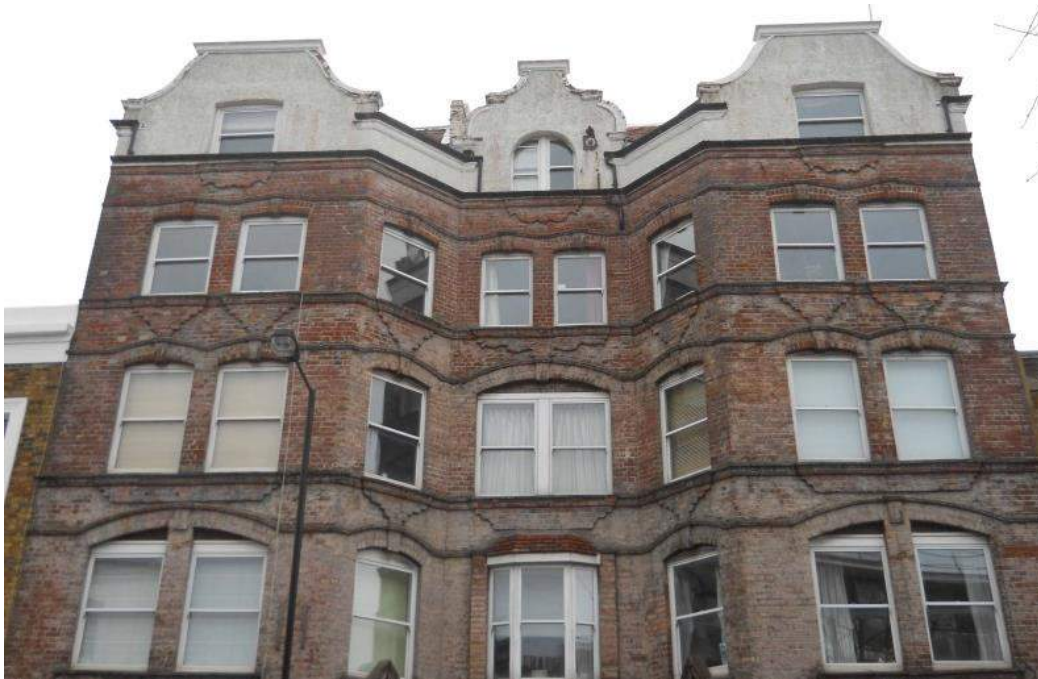
Elaborate brick detailing, no. 112 Blythe Road.
