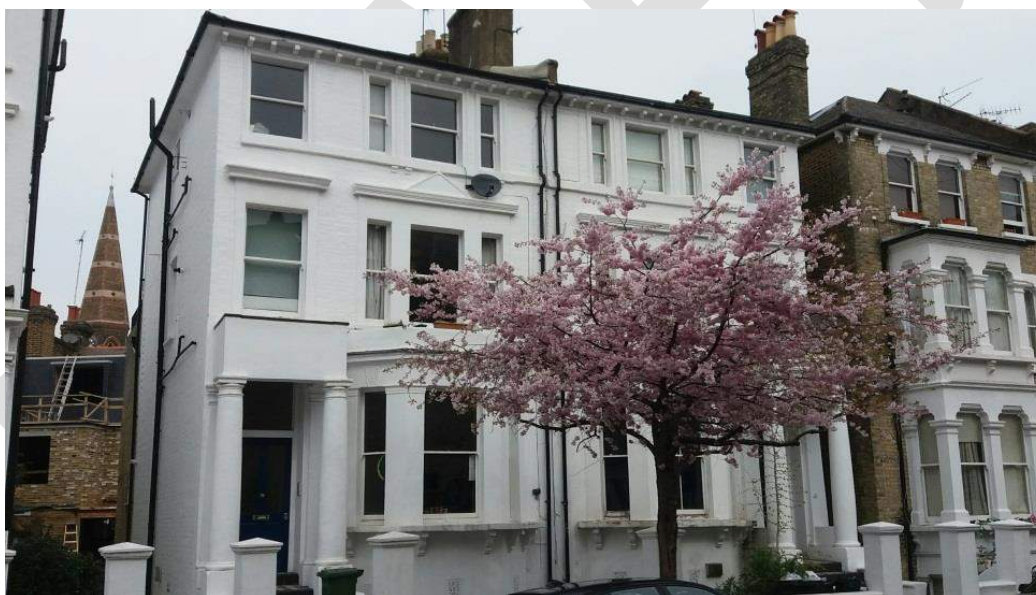
Gault brick no. 61 Netherwood Road on the right and nos. 63-65 centre ground. A glimpsed view of St. Simon's Church spire on the left.
