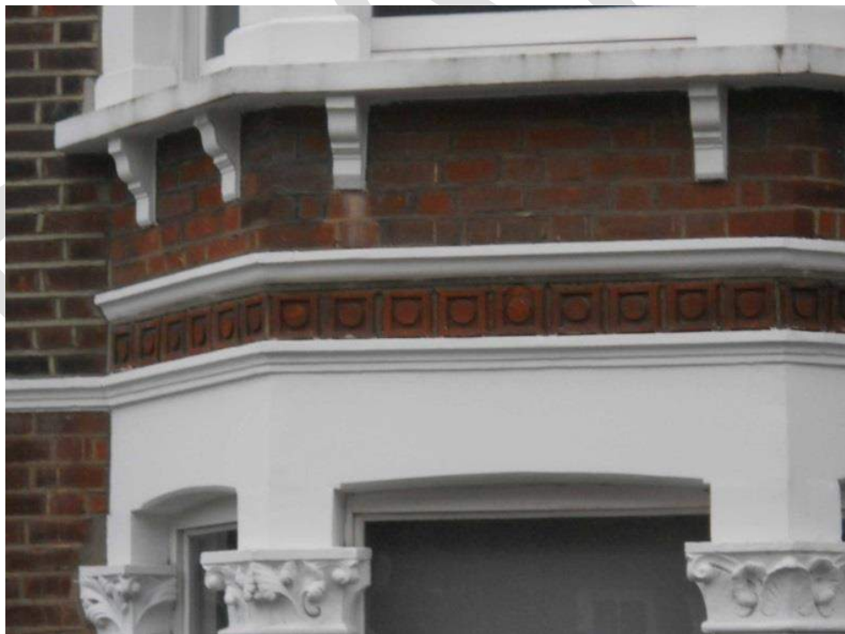
Distinctive moulded brick pattern on Nos. 69 to 83 Bolingbroke Road.
