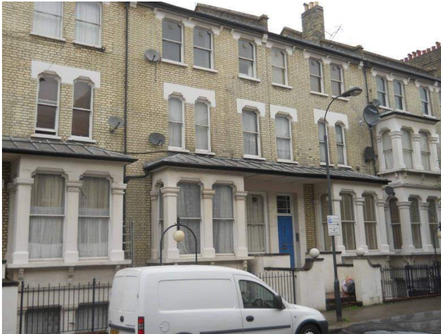
Lakeside Road, gault bricks and stucco bays found on Nos. 32-106 and 43-97.
