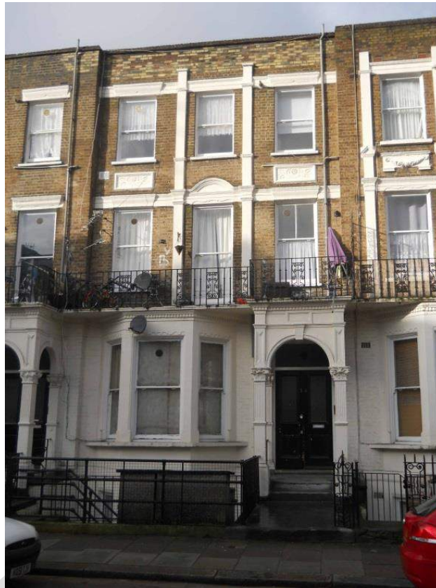
Hazlitt Road. Missing cornices diminish the decorative composition.
