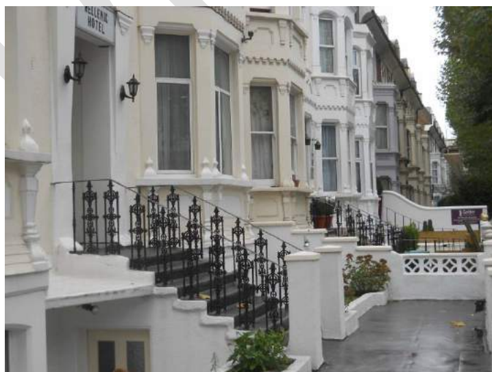
Nos. 77 to 85 Shepherds Bush Road have vase like pilasters under the sills and finials above. Ornate railings remain on some.
