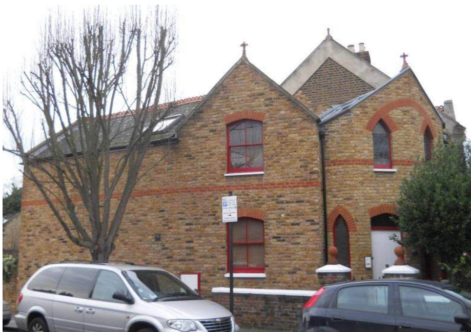
No. 1 Fielding Road turning onto Masbro Road. Attractive red brick soldier courses in window arches and string courses.
