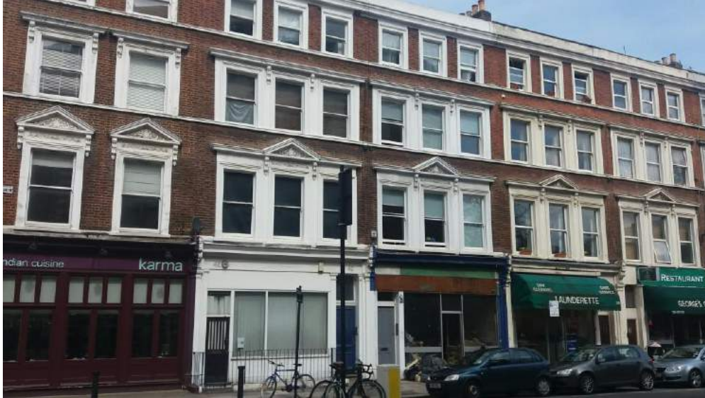
Original shop surrounds are largely intact. Nos. 2-12 Maclise Road.
