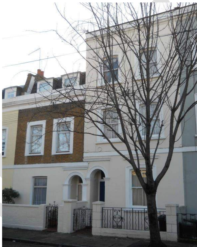
Nos. 28 (right) and 30 Milson Road.
