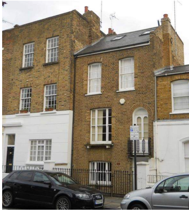
Juliet balcony provides canopy, No. 54 Masbro Road.
