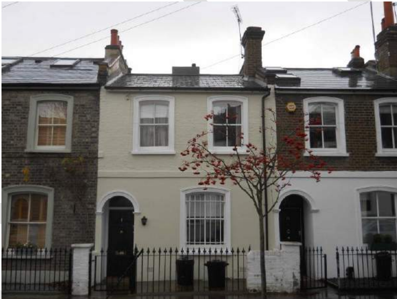
The raised ridge on the roofs to the left and right of the picture accommodates a loft extension. Faroe Road.
