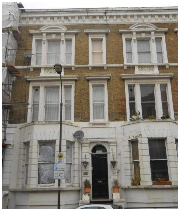
Stucco ornamentation, Nos. 2a to 24 Lakeside Road.
