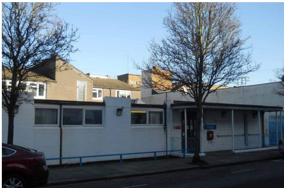
Health Centre Milson Road, an opportunity site.
