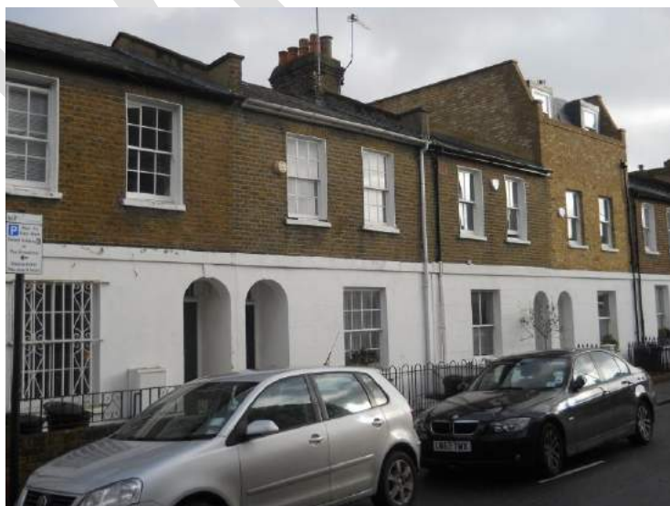
No.49 Milson Road. Prominent additional floors have disrupted the consistency of the terrace.
