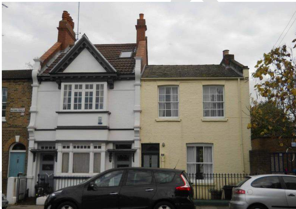
Unusual full height pilasters, No. 42 Masbro Road.
