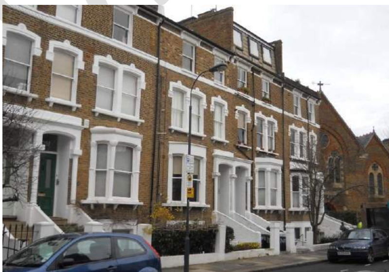
Conspicuous mansard roof on the north side of Fielding Road.
