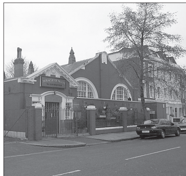
Former Post Office Sorting Office, Loftus Road
