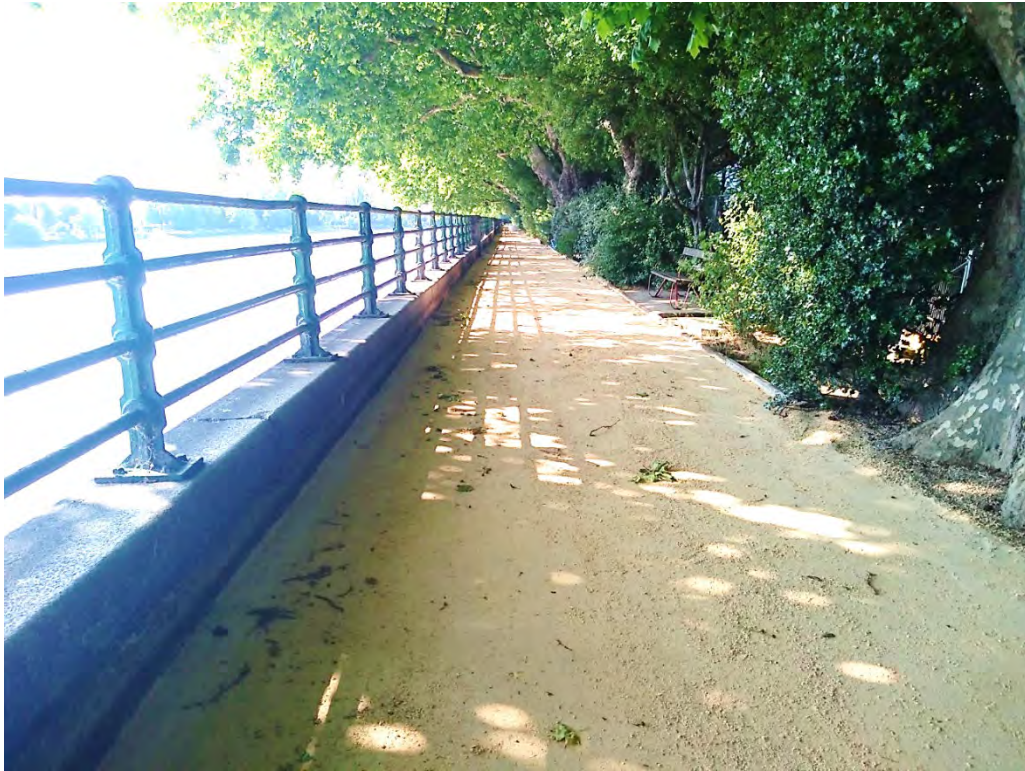
Figure 12: Bishops Park – Footpath resurfacing along the riverside. Previous macadam surface was de-paved and replaced with a self-binding aggregate material.
