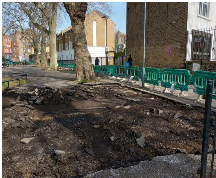
Figure 17: Footpath resurfacing of north area – ‘de-pave’ of macadam surface and reinstatement with self-binding aggregate at Eel Brook Common
