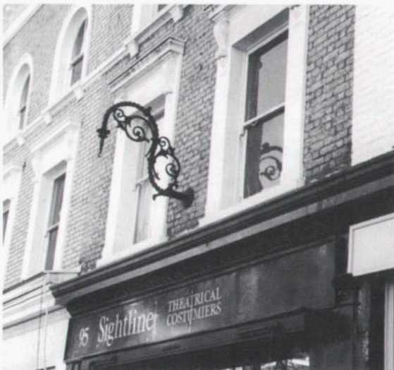
Hanging bracket and traditionally detailed fascia intact on No. 95
