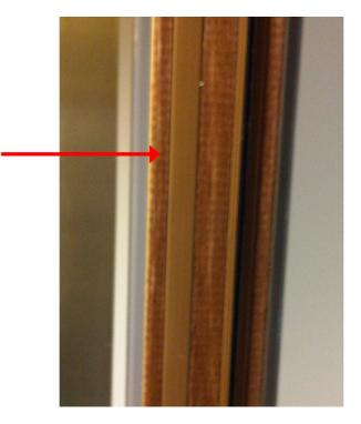
**Smoke brushes** – these do the same job as smoke seals but in a slightly different way. Make sure they are not painted over, worn or missing in parts
