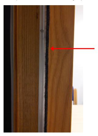
**Self-closing device** – these make sure that the door closes when opened, it should be smooth without the door banging loudly against the frame (this will cause damage in the longer term). The self-closer below is the most common, but they can be fitted into the frame so may not be obvious. The key test is whether the door closes independently and snugly into it's frame.
