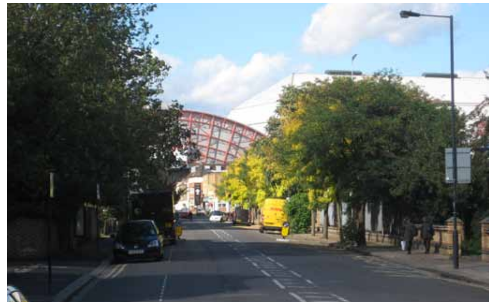
Figure 33: Photograph of Seagrave Road Carpark boundary with the OA along Seagrave road
