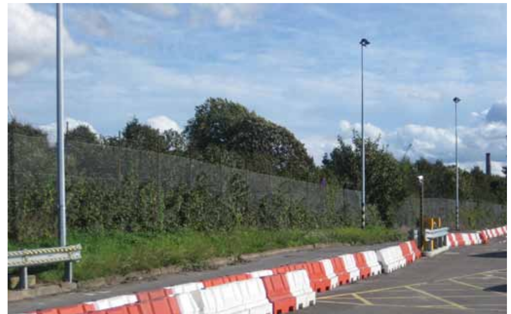
Figure 38: Photograph of Seagrave Road Carpark boundary with the OA
