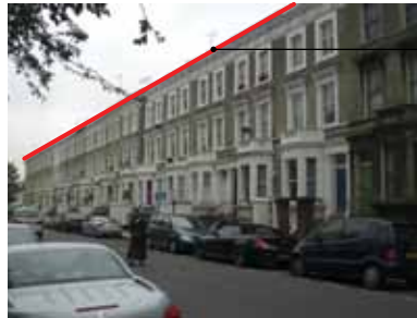
strong, consistent parapet line with nothing visible above it
