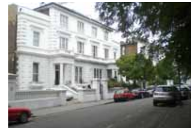
Figure 1.365: White Stuccoed villas at The Boltons
