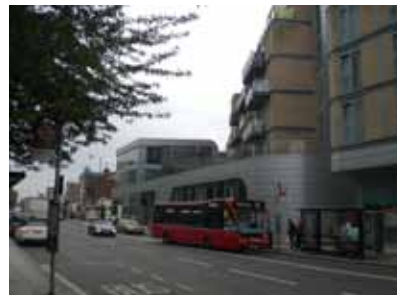
Figure 1.155: Primary Street: North End Road
