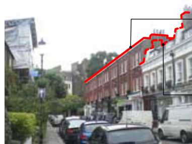
simple, consistent parapet line roofscape articulated by dormer windows and mansard roofs
