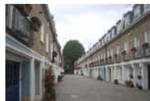
Figure 1.350: 2 storey mews houses
