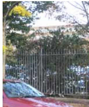
Figure 1.74: Railings on Seagrave Road
