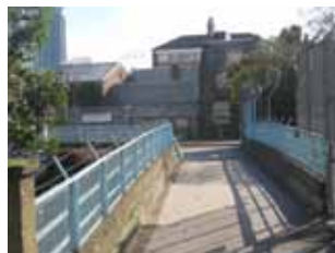
Figure 1.34: Footbridge across the railway
