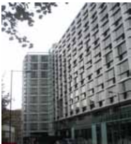
Figure 1.249: 10 storey Think Building
