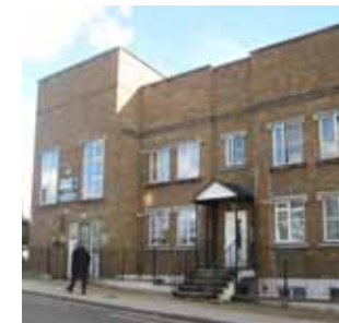
Figure 1.60: Block of flats on Lillie Road
