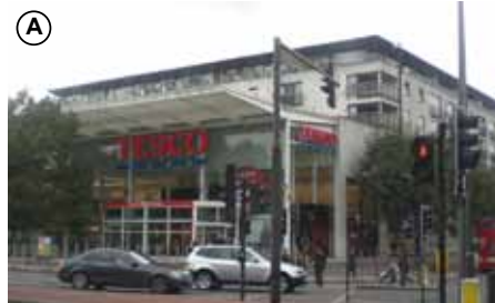
Figure 1.222: Local Landmark: The location of the Tesco supermarket on the highly prominent junction between West Cromwell Road and Warwick Road gives it significance as a local landmark.
