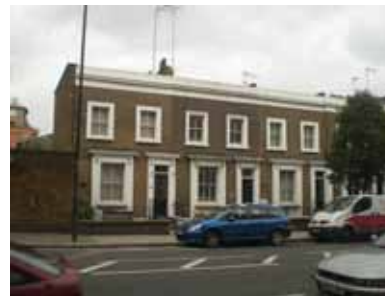
Figure 1.251: 2 storey terraced houses on Warwick Road
