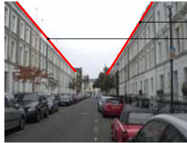
simple, consistent parapet lines with nothing visible above them on both sides of the street
