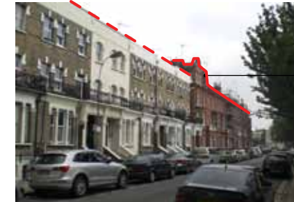
mid terrace variation in roofscape
