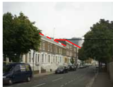
mid terrace variation in roofscape
