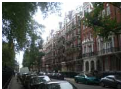
Figure 1.292: 5.5 storey buildings overlooking Braham Square communal gardens
