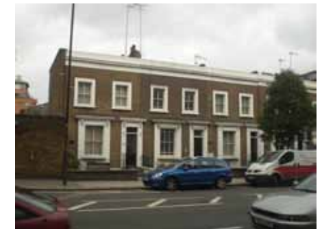
Figure 1.236: A low rise terrace in the area
