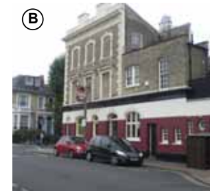
Figure 1.80: Local Landmark: The Harwood Arms pub
