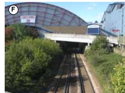
Figure 1.53: Distant Landmarks: view of Earl's Court 2 from Lillie Road railway bridge
