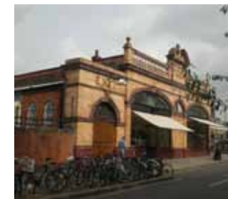
Figure 1.178: Barons Court Station
