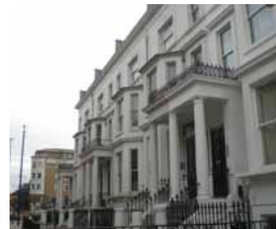
Figure 1.235: Terraced town houses in the area
