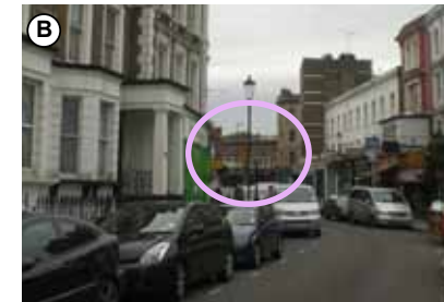
Figure 1.256: Local Landmark: Earl's Court Station acts as a point of reference which terminates local views
