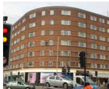
Figure 1.192: An example of a perimeter block in the area
