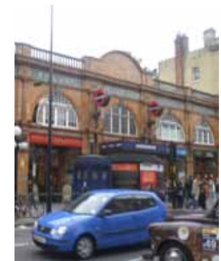
Figure 1.309: Earl's Court Station
