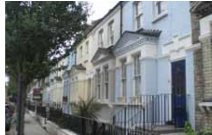
Figure 1.161: 2 storey low rise terraces
