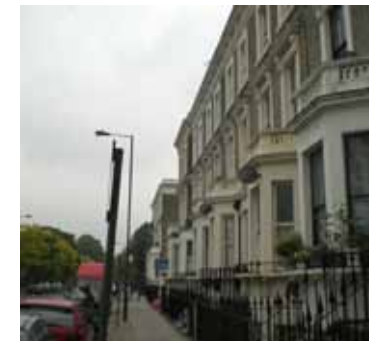
Figure 1.69: The 3.5 storey town houses
