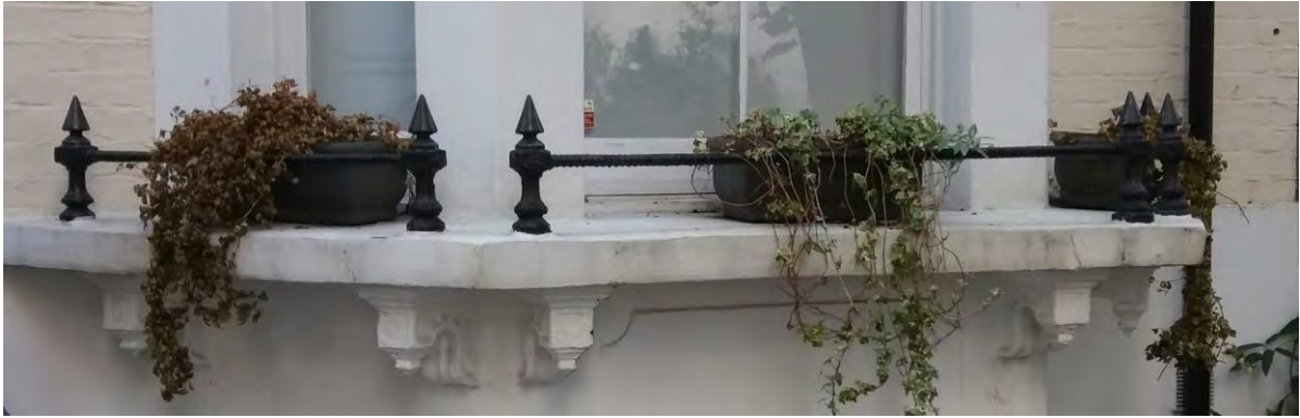
Original wrought iron window sill castings.
