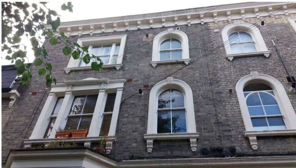
Deep cornices with moulded modillions. An original feature of Nos. 2-10 Barclay Road. Missing on Nos. 2 & 4.
