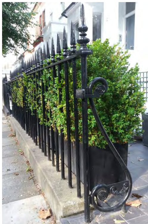
Spear type railings and iron backstays with integral boot scrapers.
