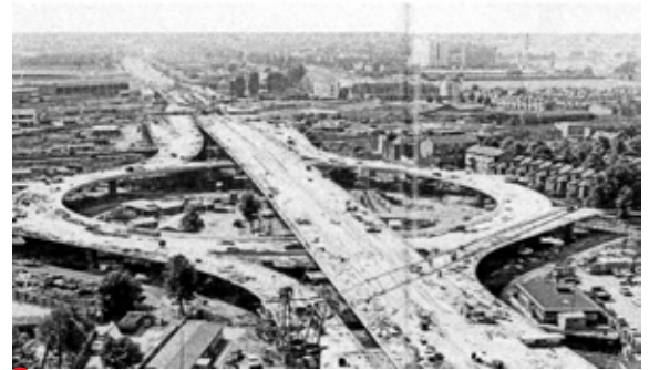
① Construction of the Westway (1960s)
