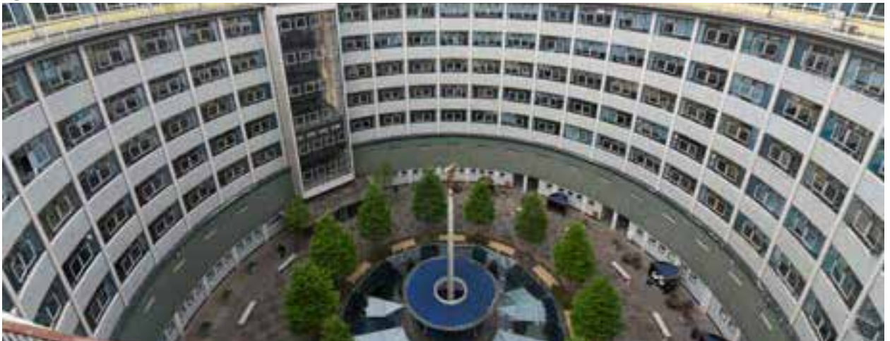
Figure 3.41: BBC TV Centre, Inner courtyard
