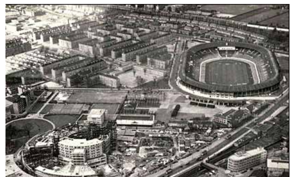
④ BBC TV Centre under construction
