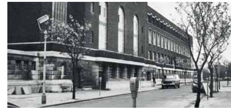
West Elevation looking south down Nigel Playfair Avenue
