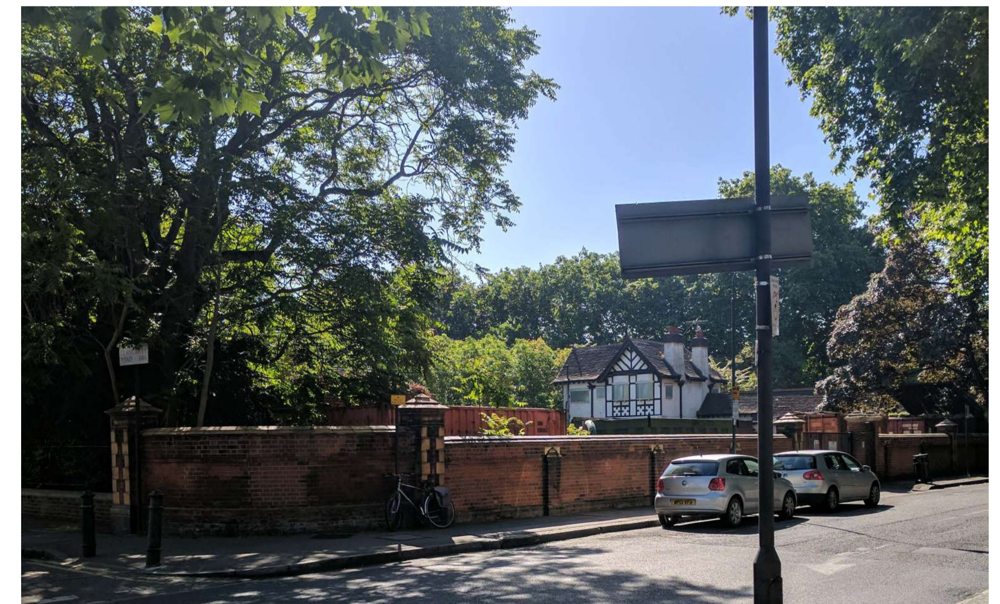
3. View of the site on approach from Peterborough Road
