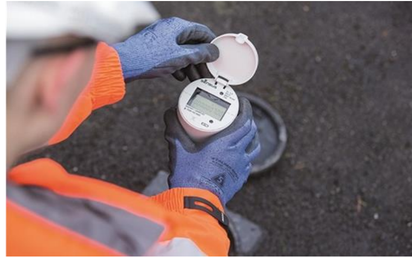
Image 4: Fitting a water meter
