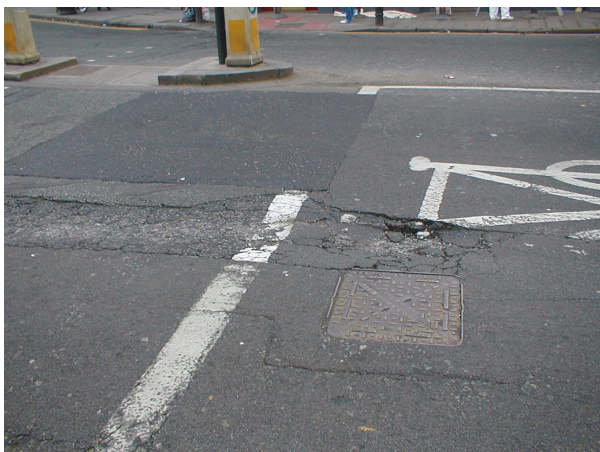
Example of Utility works defect
