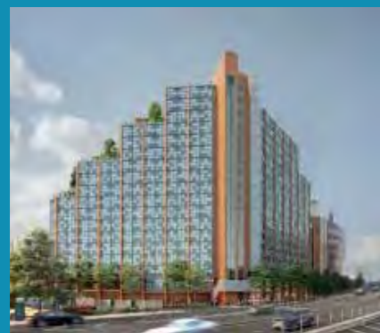
161 Talgarth Road - Under Construction
