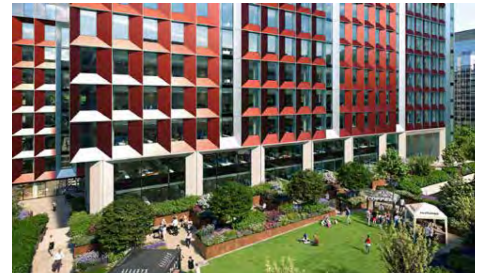
Podium Gardens behind 245 Hammersmith Road
