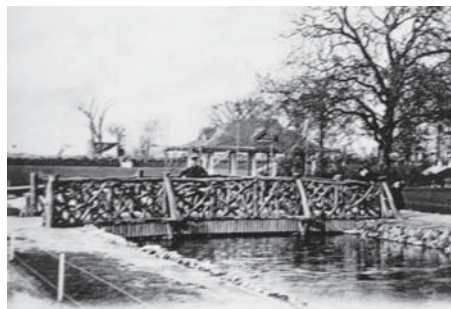
Rustic timber bridge c. 1900
